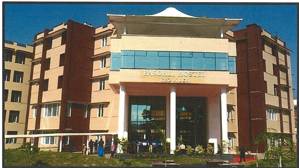
A view of Basohli Boys Hostel at SMVDU
