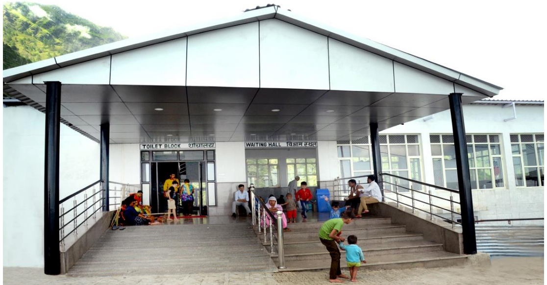
The biggest Toilet Complex commissioned at Adhkuwari.
