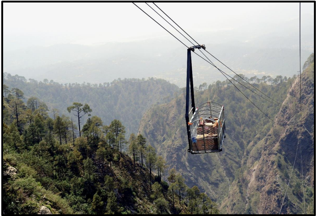
A view of the Siar Dabri-Bhawan Material Ropeway
